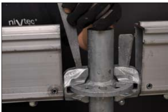
attach wedge head to rosette
