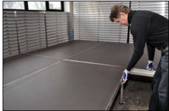
hook tongue profile into groove profile
