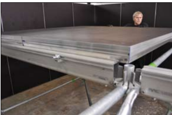
put on platforms and lock connections
