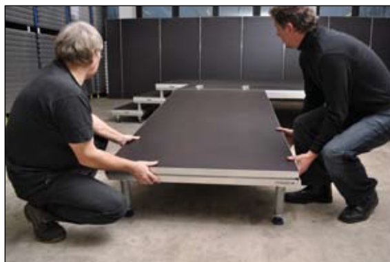
mount 2 legs and hook platform on stage
